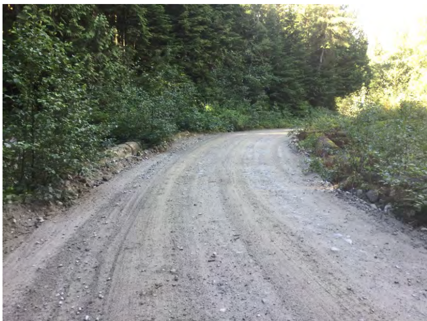
Approach from Right Bank when facing downstream
